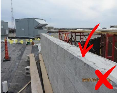
**Wall is not protected at the top...even grouted solid walls must be protected.**
