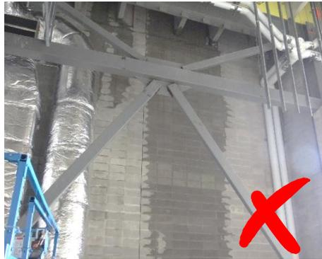
**Water has entered from the top or is washing down the face of the interior CMU...this will cause the AVB to fail**
