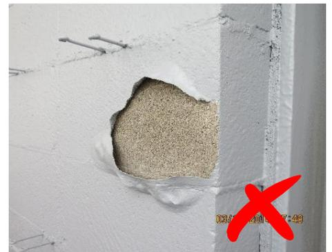
**Moisture has driven to the exterior face of the CMU, pushing the membrane off the wall.**
