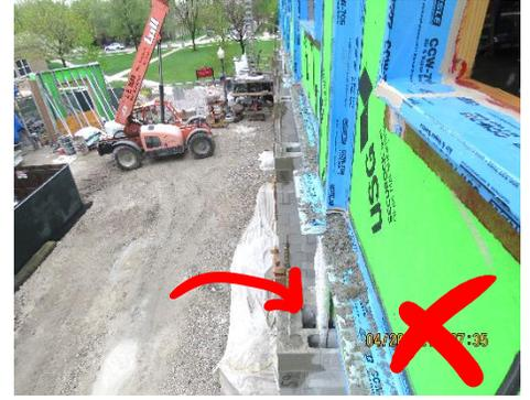
**The wall as it is installed at the end of the day must be covered.**
