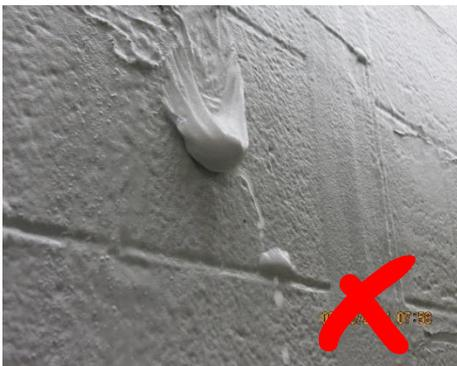
**A lot of water in the CMU...causes the membrane to fill with water behind the membrane.**
